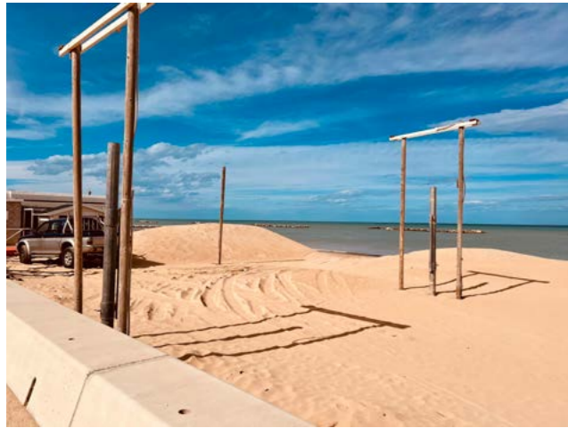
Fig. 10-11 Examples of artificial dunes constructed to protect against storm surges, Francavilla al Mare, Chieti. Photo by K. Di Chello © 2024
